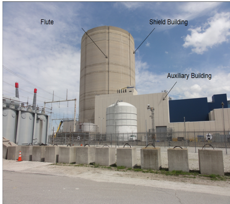
Figure 2: Davis-Besse Shield Building
