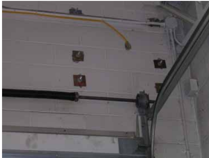
Figure 4 – Through-bolts with backing plates
