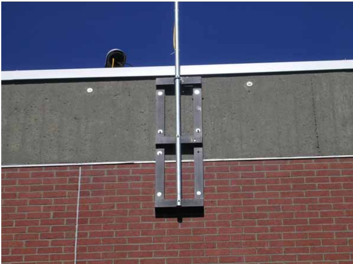
Figure 1 - Flush Mount used on buildings with small roof overhang
