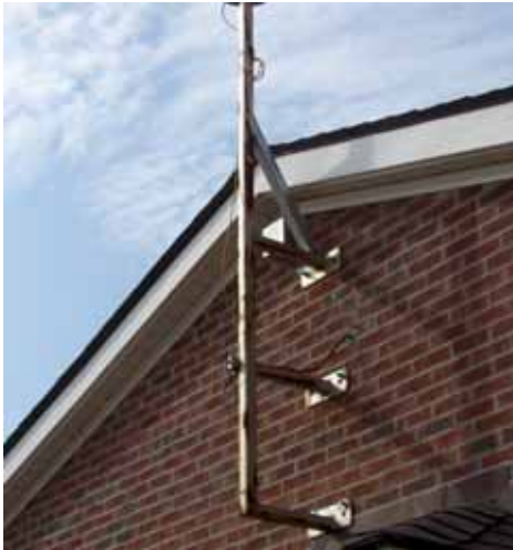
Figure 2 - Outrigger Mount
