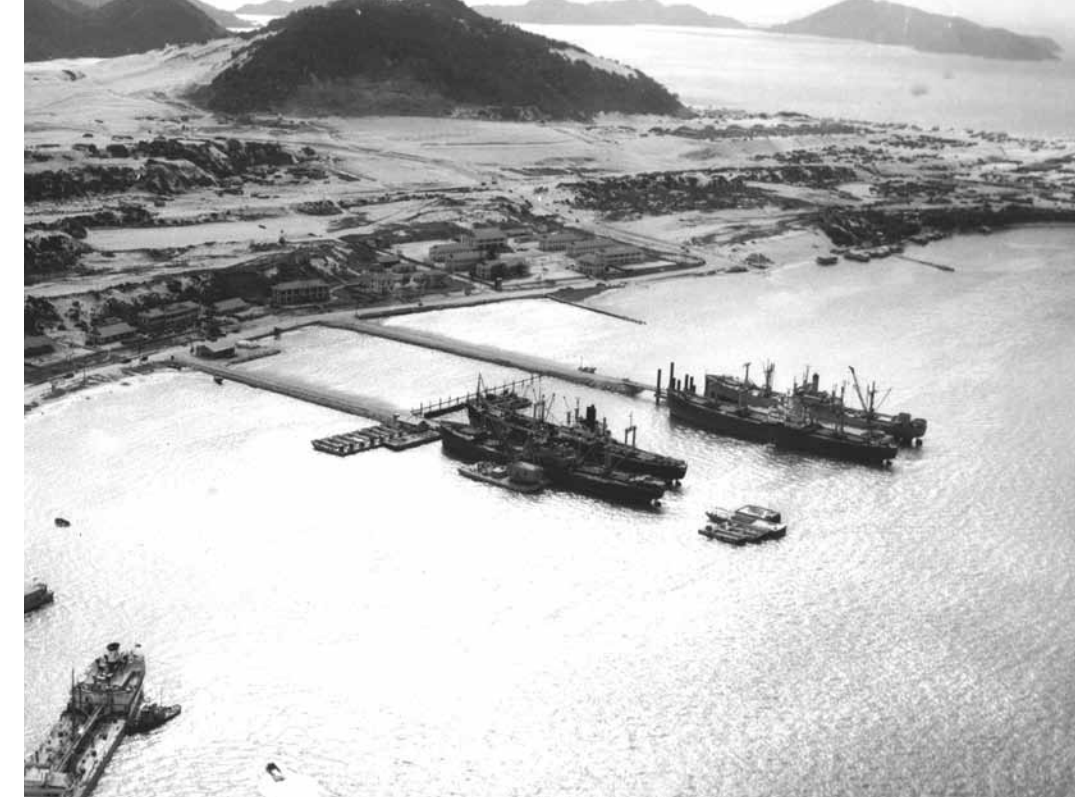
DeLong floating piers like this one at Cam Rahn Bay made the development of deep-draft ports in South Vietnam possible.
