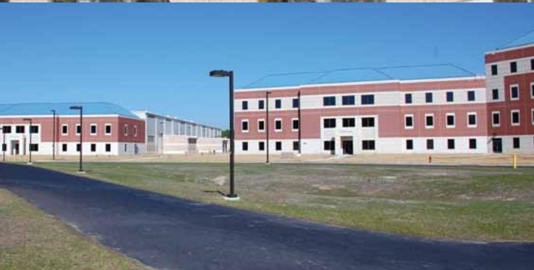
Above: The new Army Ordnance School has 15 training facilities, like these, with training bays. (Photo by Albert Cruz, BRAC Construction Office)
