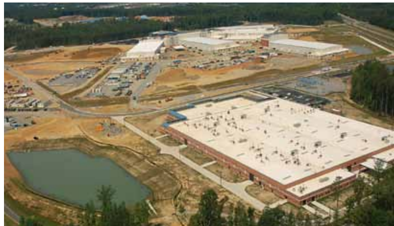
The 16th Ordnance Battalion has begun training at the Tactical Support Equipment Directorate’s new building, lower right, at the Ordnance School campus at Fort Lee, Virginia.
