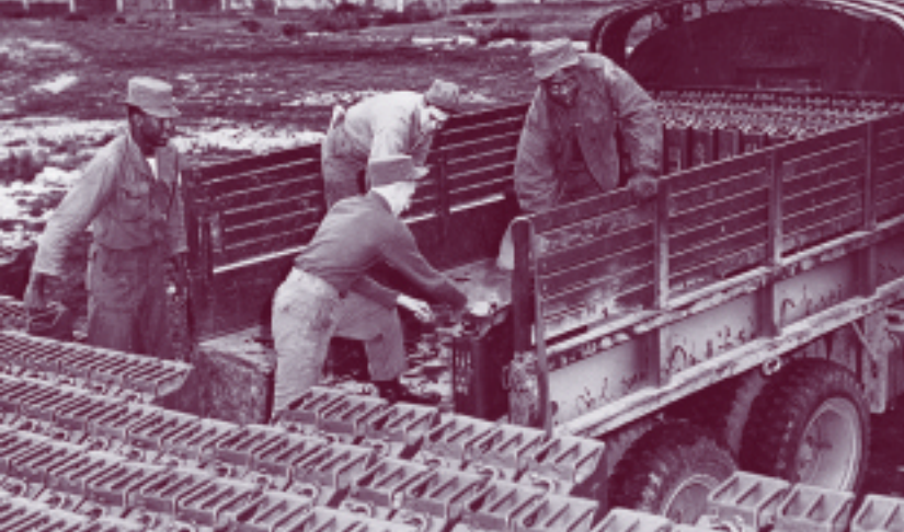
Soldiers load some of the approximately 20 million 5-gallon cans that were used to refuel vehicles during World War II.
