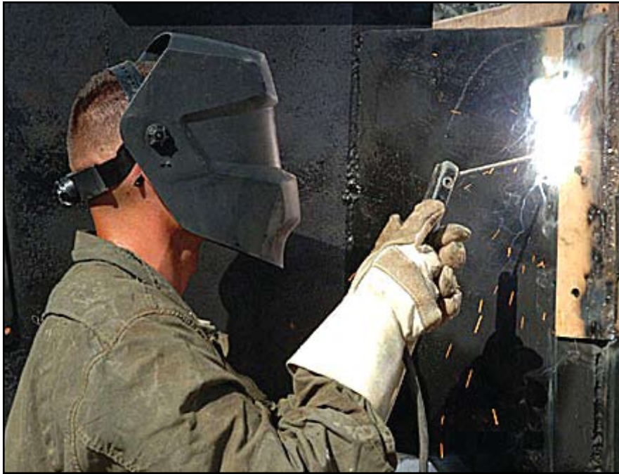
Welders from the 27th Brigade Support Battalion, 4th Brigade Combat Team, 1st Cavalry Division, deployed to Forward Operating Base Marez, Iraq, fabricated the first up-armored pickup truck for the Iraqi police. The truck provides security for Iraqi policemen manning checkpoints. The welders' success led to a tasking to create four more up-armored pickups for the police. (Photo by PFC Bradley J. Clark, 4th Infantry Division PAO)
