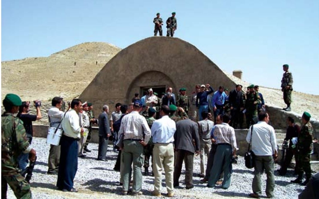
Members of the Afghanistan National Army general staff inspect a renovated ammunition bunker at the opening ceremony of the Khairabad Ammunition Depot.
