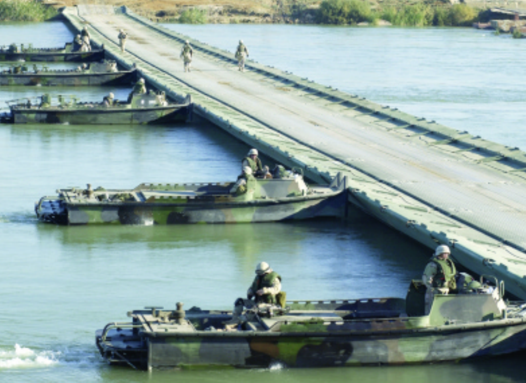
Soldiers of the 502d Engineer Company, 565th Engineer Battalion, 130th Engineer Brigade, from Hanau, Germany, position their bridge-erection boats against the current as they remove a Mabey-Johnson float bridge from the Euphrates River near Al Qaim, Iraq. The float bridge provided a vital crossing point for the people in the area after bombing by insurgents rendered the original bridge unusable for foot or vehicle traffic. Thirty-five soldiers dismantled the two land spans and seven floating spans of the bridge in November and moved them to Assydnia, which is near Forward Operating Base Anaconda.
