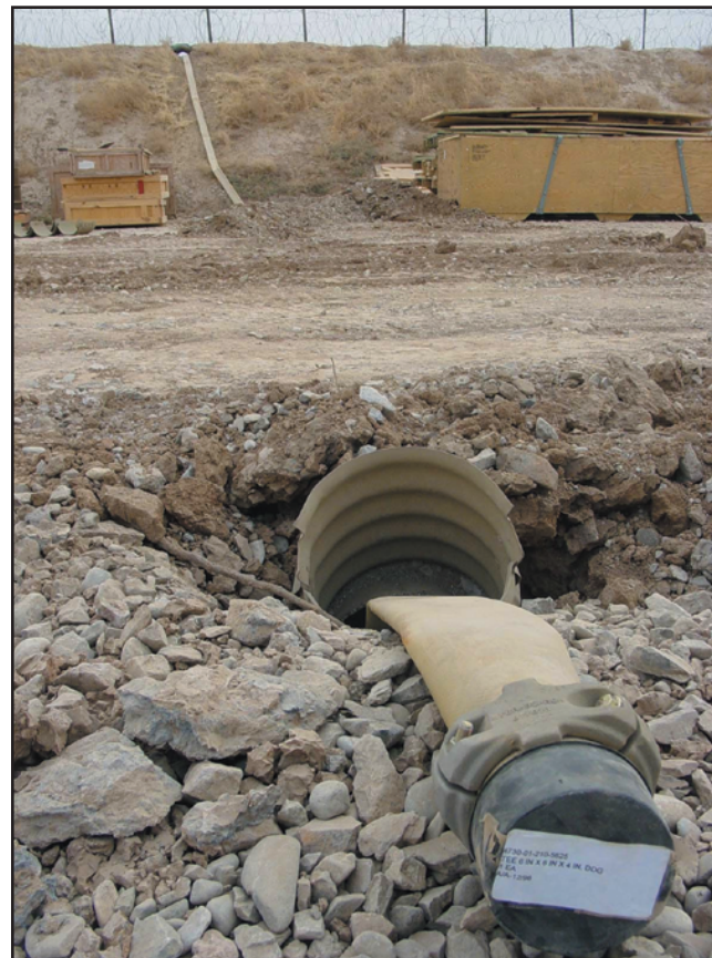
□ The assault hoseline can transfer fuel from an Uzbekistan Ministry of Defense fuel farm to a U.S. Army fuel farm when necessary.
