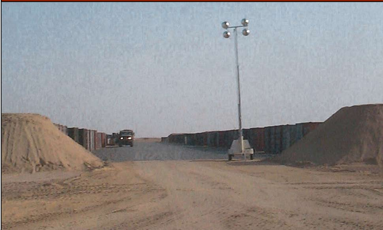
A barricaded ammunition storage pad at Camp Arifjan, Kuwait.
