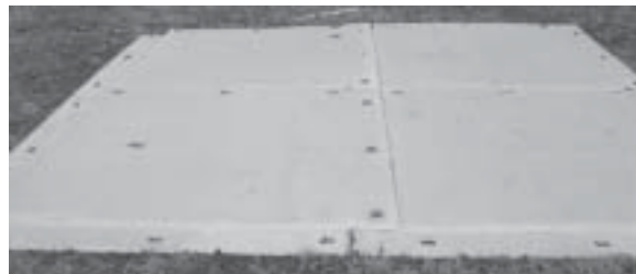
□ Fiberglass-reinforced mats are bolted together to provide a resilient road surface.
