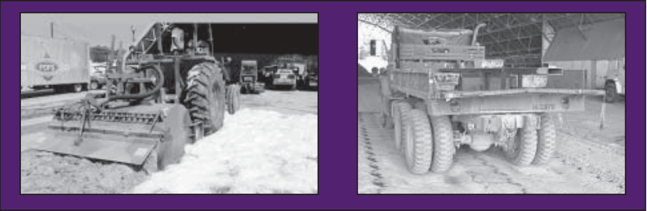
□ Left, geofibers are mixed with sand to create a stable base for a resin-modified emulsion or emulsified asphalt surface. Right, hexagonal mats are designed for quick installation to create parking areas and access roads.
