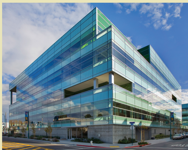
JBEI Research Facility. JBEI researchers are located at a single site in Emeryville, California. [Photo by Roy Kaltschmidt, Lawrence Berkeley National Laboratory]
