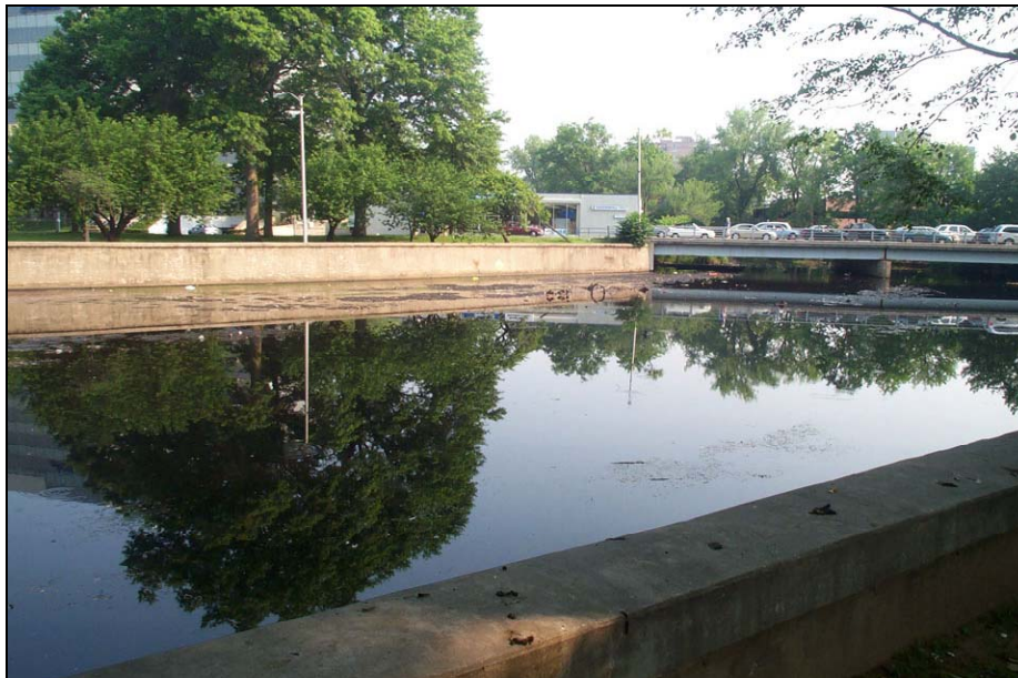
Plate 1. Mill Pond in downtown Stamford, CT, showing concrete retaining walls lining the pond.
