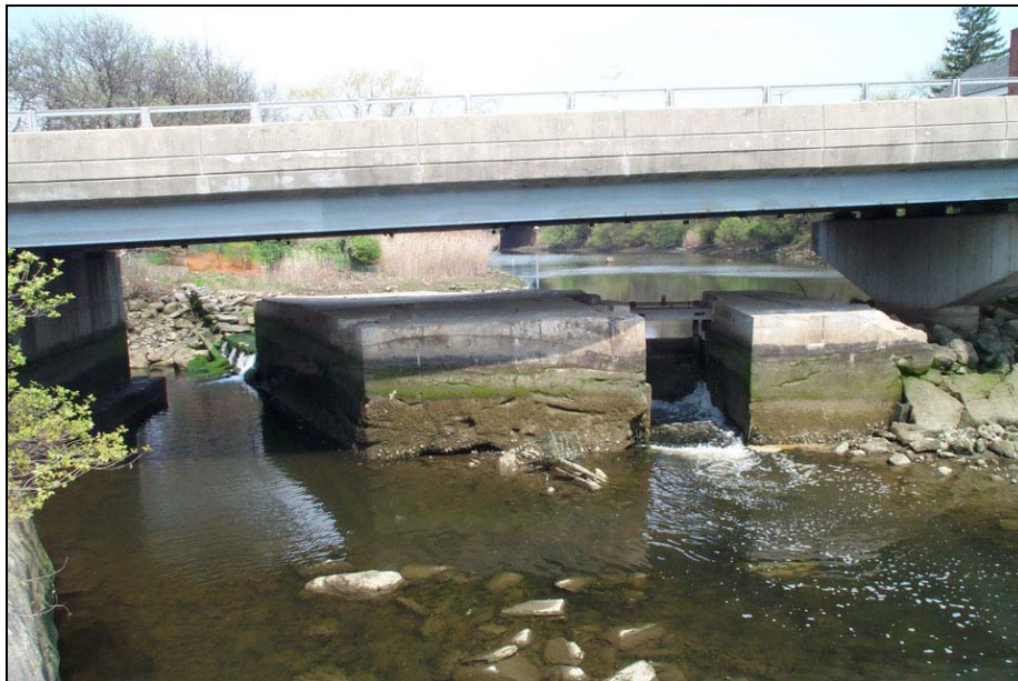
Plate 9. Concrete blocks under Pulaski Street Bridge.
