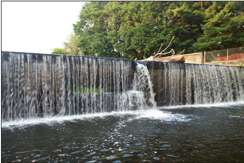
Plate 6. Sheet flow over the Main Street Dam.
