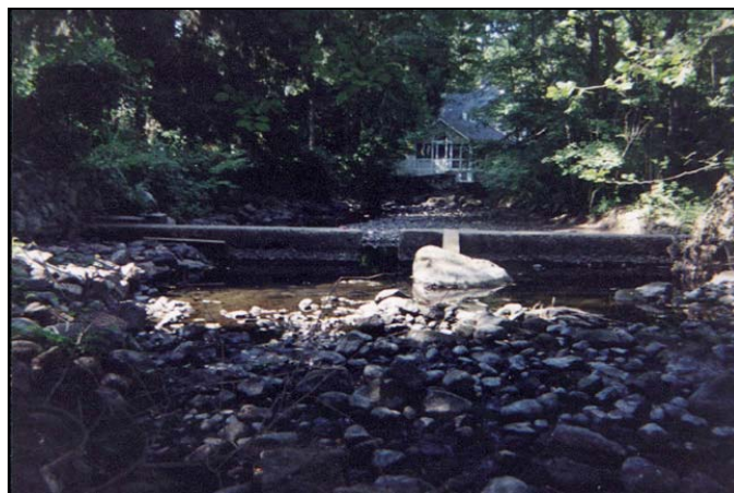
Dam 2: General Electric, 260 Long Ridge Road, river mile 4.88. This dam has a notch in the center allowing fish passage.
