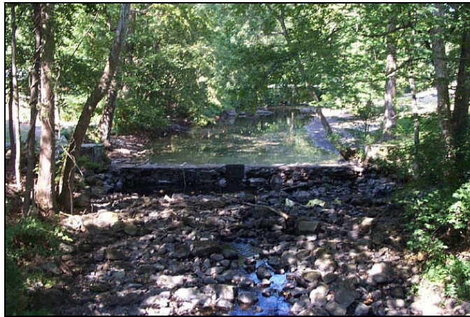
Dam 7: Merritt Parkway, river mile 6.05. This dam does not currently allow fish passage, but there is a gate in the center of the dam that could easily be opened to restore fish passage.
