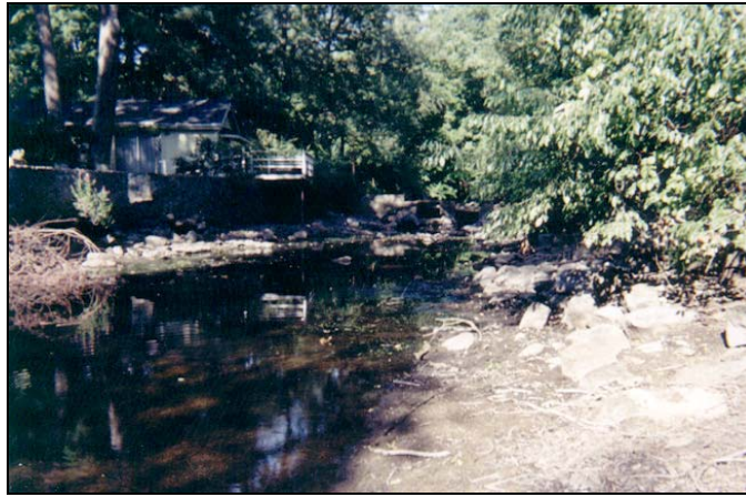
Dam 4: North of Arden Lane, river mile 5.25. Similar to Dam 3 in structure. Base of dam blocks fish passage.
