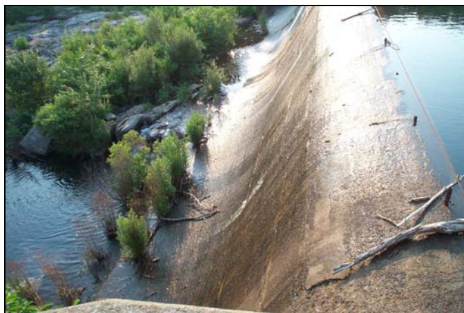
Dam 8: North Stamford Dam, river mile 8.13. No fish passage.
