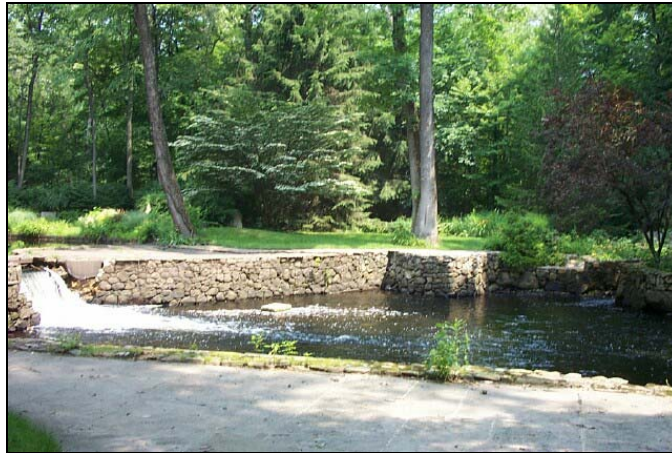
Dam 6: Hunting Lane, river mile 5.49. This dam is similar in structure to Dam 5, with a side channel allowing fish passage.
