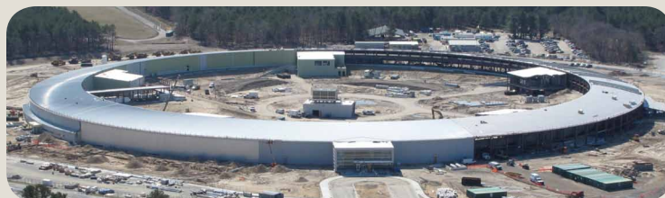
Fig. C1. NSLS-II under construction and ~50% complete on March 25, 2011. The new facility will produce photon beams with a brightness and coherence unsurpassed by any synchrotron worldwide and will support a wide range of experiments in the biological and physical sciences. [Courtesy of Brookhaven National Laboratory]
