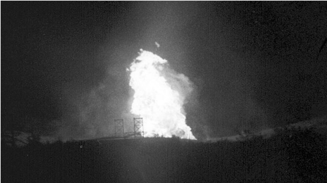
Post rupture fire – the 85-foot tall support structures for the pipeline bridges across the river are visible in lower left.
