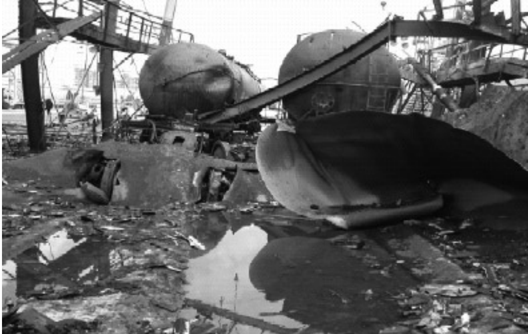
Rupture of railroad tank car in Freeport, Texas.
