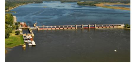
and the upper gate bay of an auxiliary lock. The main lock has the standard 110-foot-wide by 600-foot-long chamber. The average lift is 15 feet. Both the lock and the movable dam are pile-founded structures.
