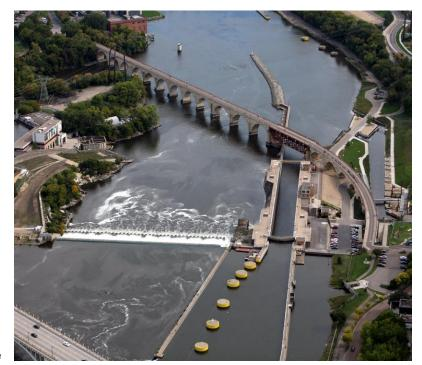
from upstream progression. Since the concrete dam was in place, the Corps only needed to construct a navigation lock. But, with a rise of 49.1 feet, the lock was the highest lift on the river and an engineering challenge costing more than \$18 million to build.
