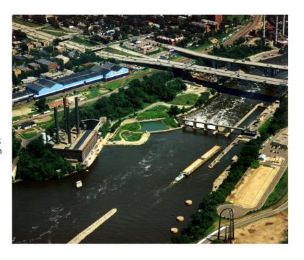
The movable dam has three Tainter gates (24 feet high by 56 feet long) and an auxiliary lock submersible Tainter gate (24 feet high by 56 feet long). Completing the dam system is a concrete non-overflow wall owned by the Corps and a short, earth embankment owned by Xcel Energy, both on the left descending bank.
