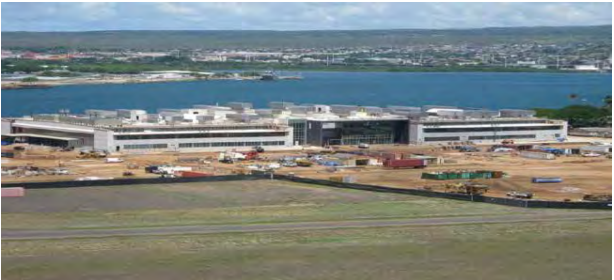
Current status of construction, August 2012.
