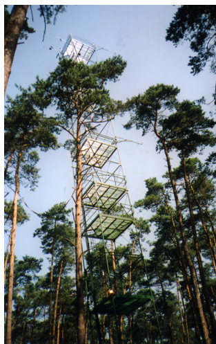
Figure 2: View of fluxtower at Brasschaat FLUXNET site
