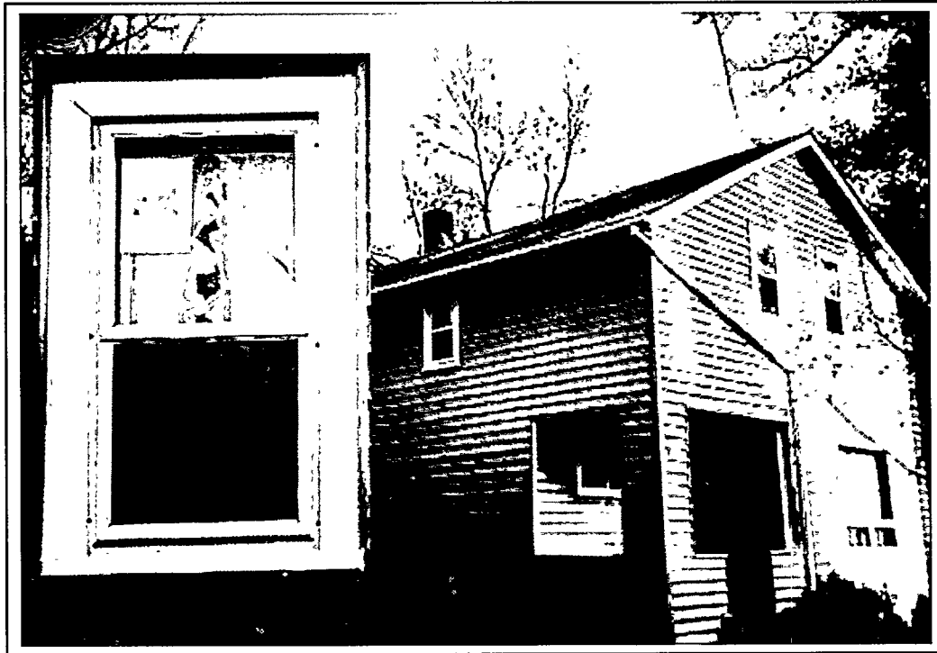
This rehabilitated home had new windows installed with HUD funds, and insulation installed with DOE funds.
