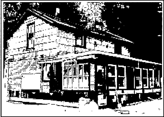
An uninsulated attic and air leakage between the porch and main structure are the main energy problems with this dwelling.
