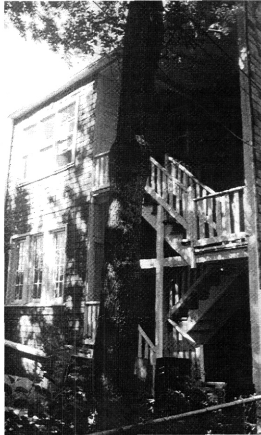
Fig. 4.5. Enclosed porches provide real challenges for Chicago multifamily contractors.
