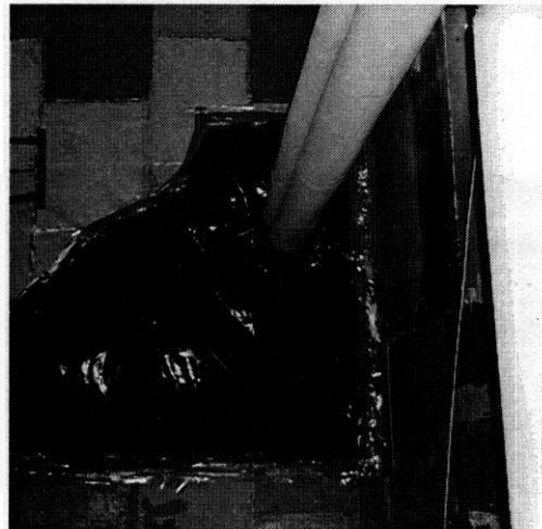
Fig. 2.11. Air sealing work completed by the building superintendent.
