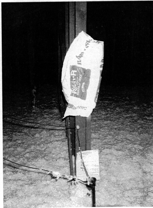
Fig. 6.33. The attic insulation job shows good, even coverage to R-38 (12 inches).
