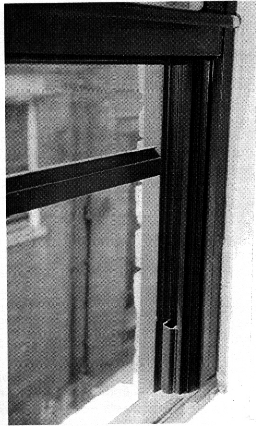
Fig. 3.9. Good-quality, double-glazed vinyl replacement windows are used in HAP's program. Installed costs are $150 to $200.
