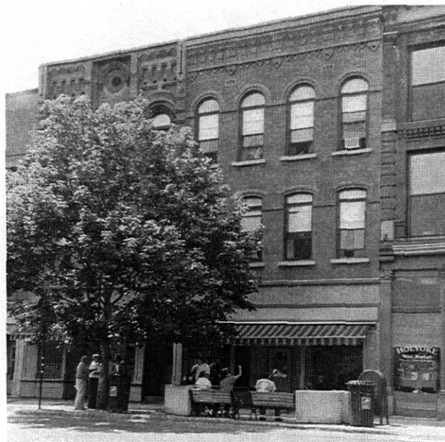
Fig. 3.11. The building at 197 High Street in Holyoke.
