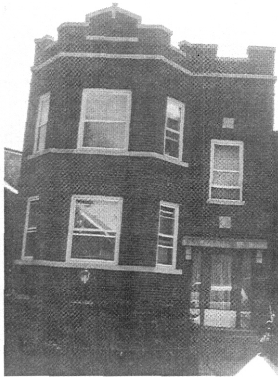
Fig. 4.4. Tenants in all five units of this three-story walkup were income-eligible.
