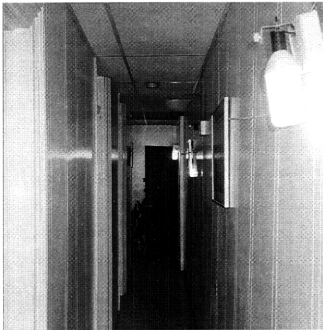
Fig. 2.6. Compact fluorescent fixtures were installed using DSM funds from Consolidated Edison. The kitchen and bathroom have energy-efficient f i r e s installed, too.
