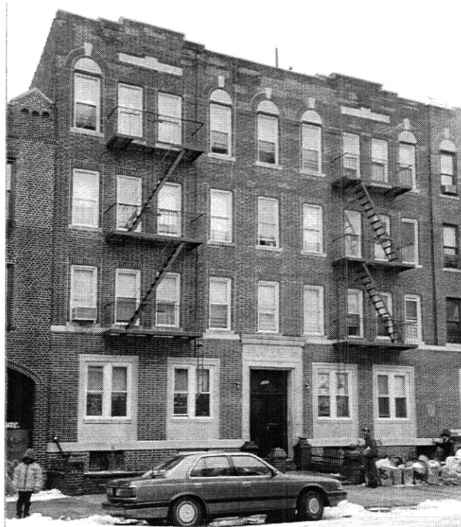
Fig. 2.15. The building at 1625 Park Place in Brooklyn.
