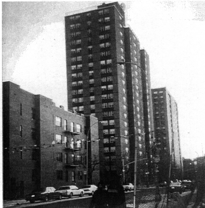
Fig. 2.18. High-rise and mid-rise buildings in the Bronx.
