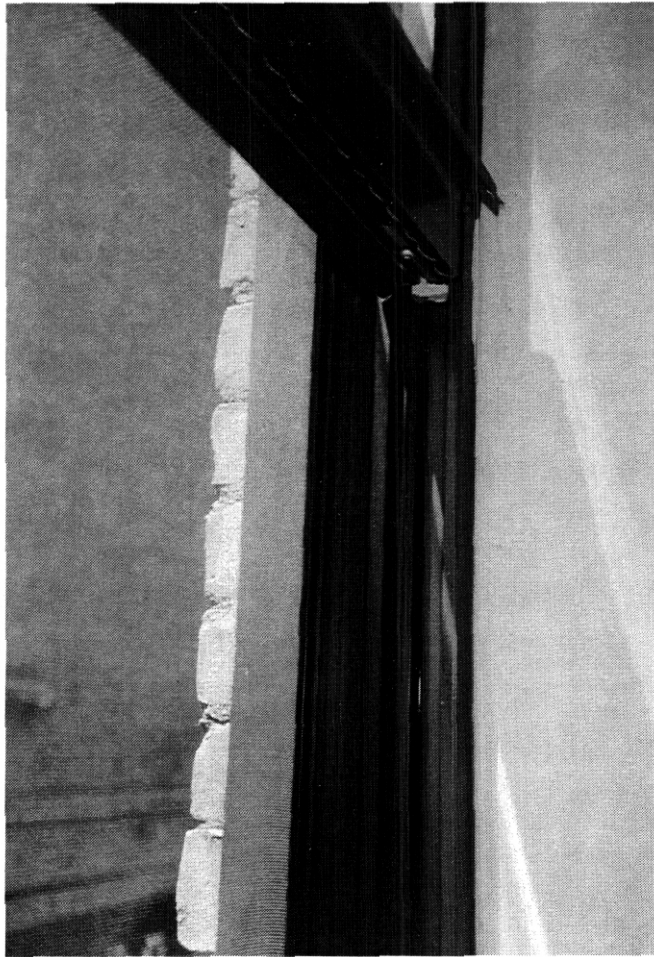
Fig. 3.12. Detail of new replacement window installed at 197 High Street.
