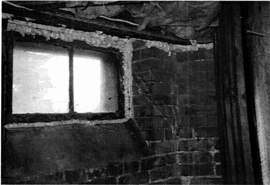
Fig. 3.15. Basement air sealing at 47—49 Vernon Street, Holyoke.
