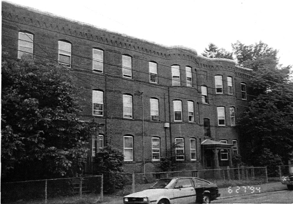
Fig. 3.13. The building at 47–49 Vernon Street in Holyoke.
