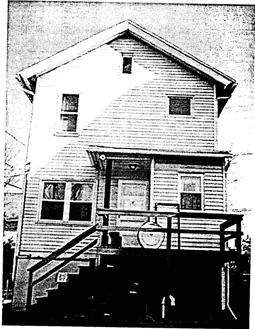
Photo 8.1 This home received storm and replacement windows.
