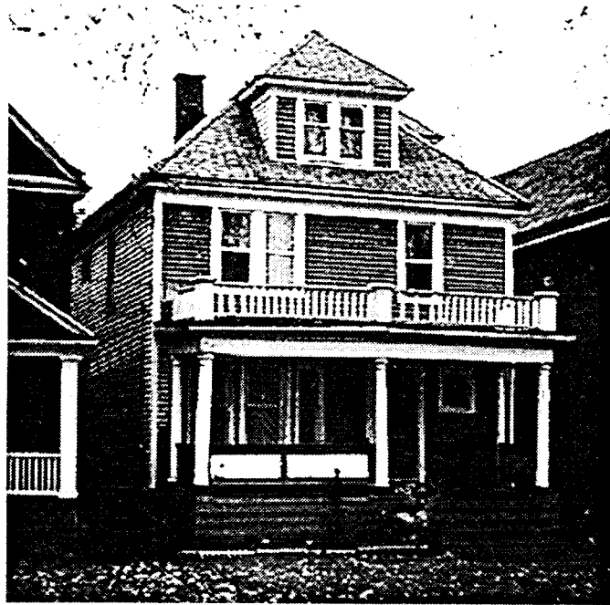
Photo 7.2 This large dwelling was weatherized by the North Buffalo CDC.
