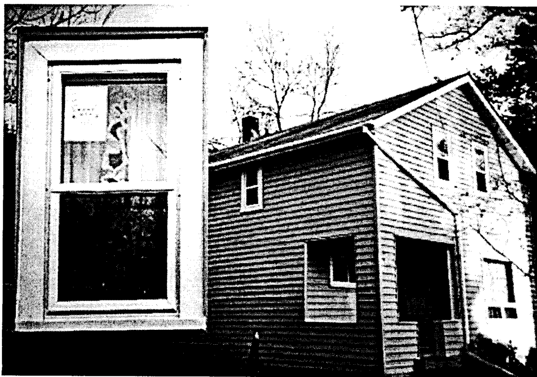
Photo 1.4 This rehabilitated home had new windows installed with HUD funds, and insulation installed with DOE funds.
