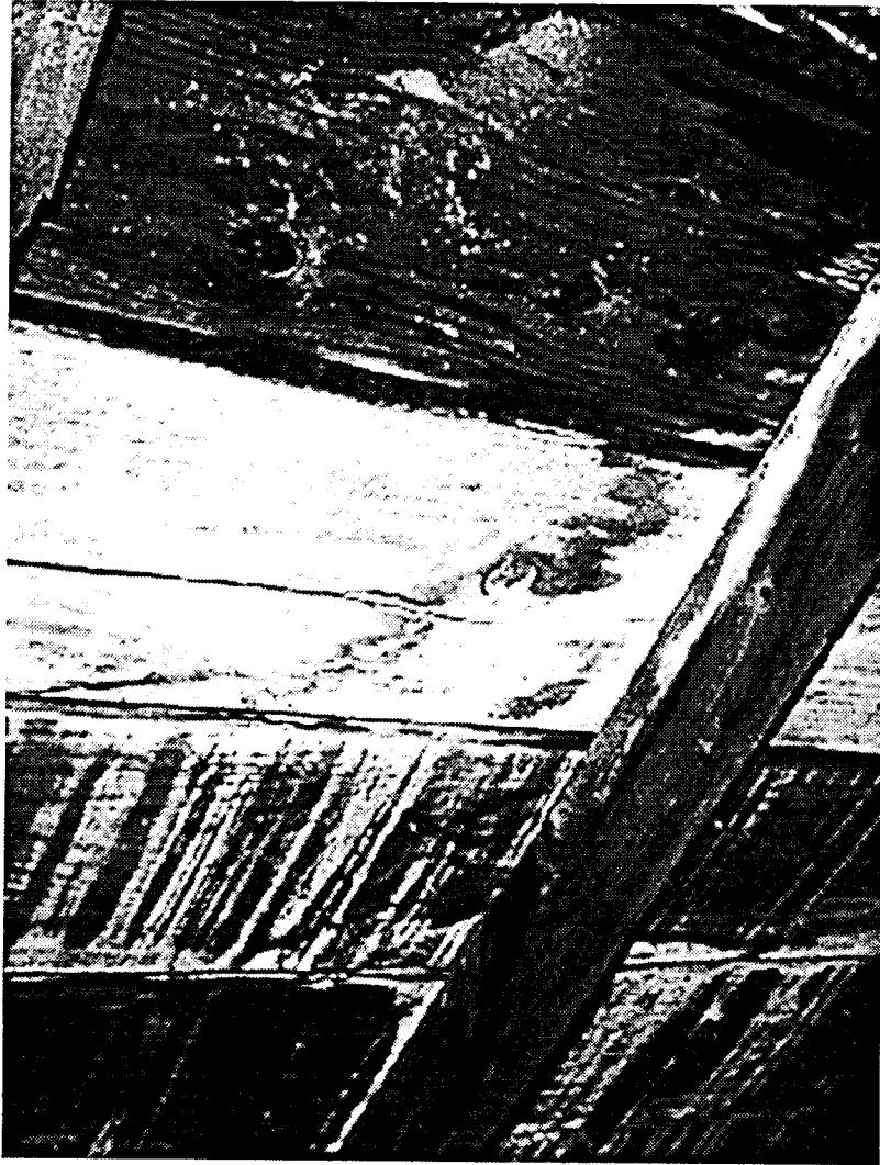
Photo 8.2 Substantial moisture damage occurred in this attic as the result of owner-installed insulation. SLHDA arrested this problem by adding attic vents, at the same time that they blew in additional cellulose insulation.
