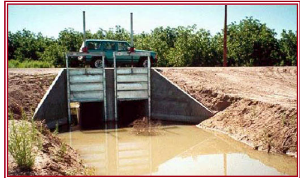
Rio Grande Wasteway at Mesilla
