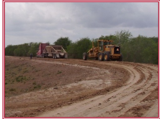
Lower Rio Grande Levee Improvements
