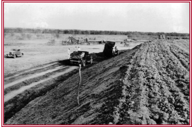
Lower Rio Grande U.S. Main Floodway
