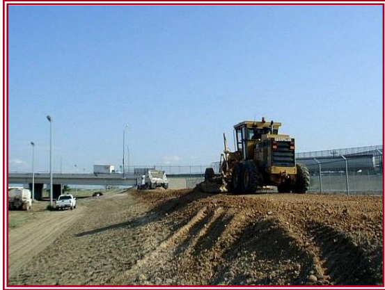
Upper Rio Grande Levee Improvements
