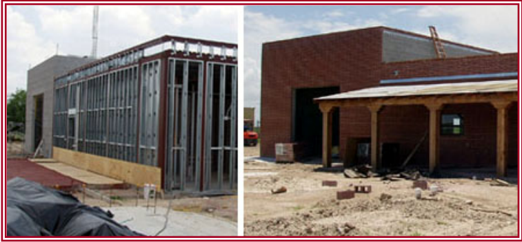
Anzalduas Administration & Maintenance Building
