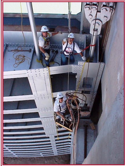
Falcon Storage Dam
