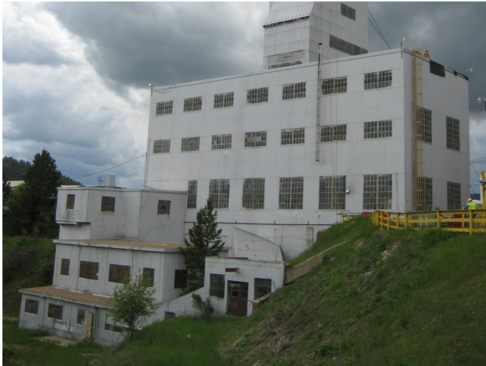
Figure A-19: Photo of Ross Crusher exterior. (HDR)
