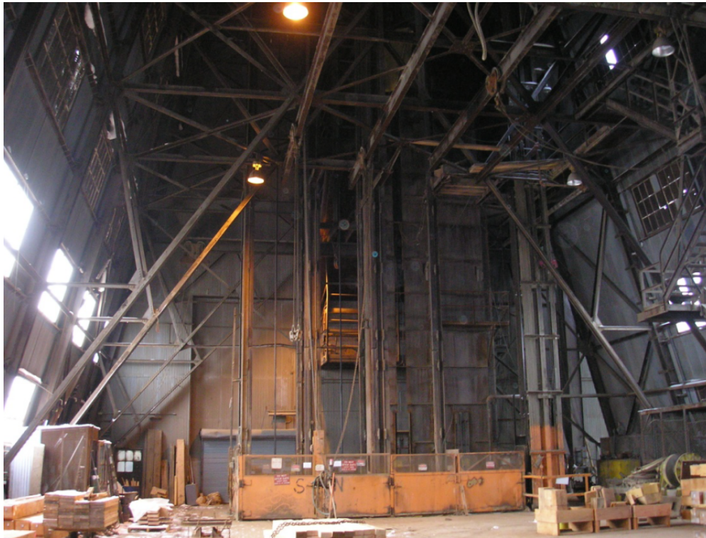
Figure A-22: Photo of Yates Headframe interior. (HDR)
