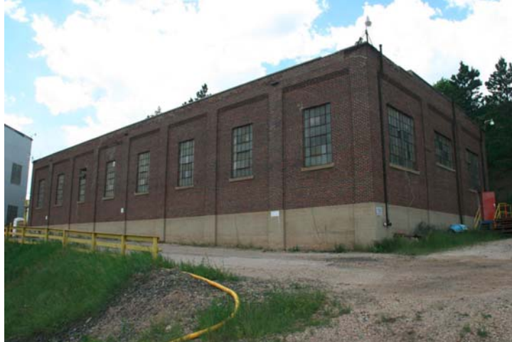
Figure 4-4: Photo of Ross Dry Exterior. [HDR]
