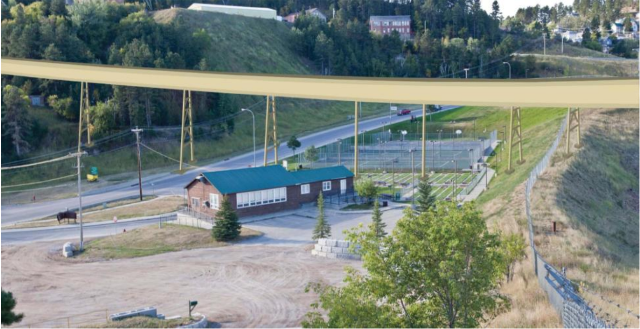
Figure 3-8: Depiction of what the pipe conveyor will look like to the Lead, SD community. [SRK, Courtesy Sanford Laboratory]
