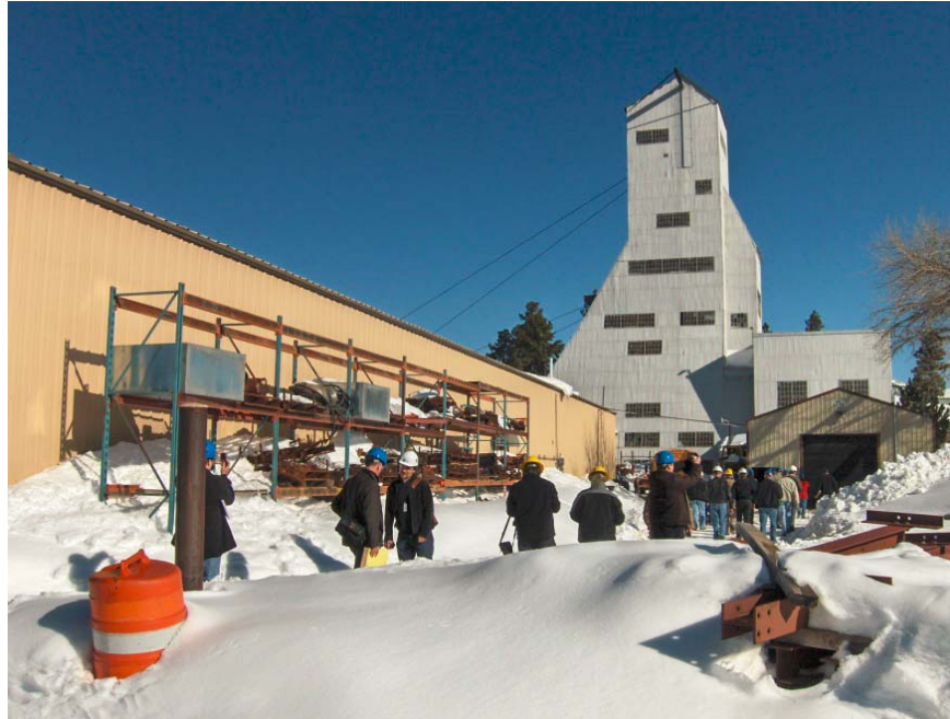
Figure 4-2: Photo of Ross Headframe. [HDR]
