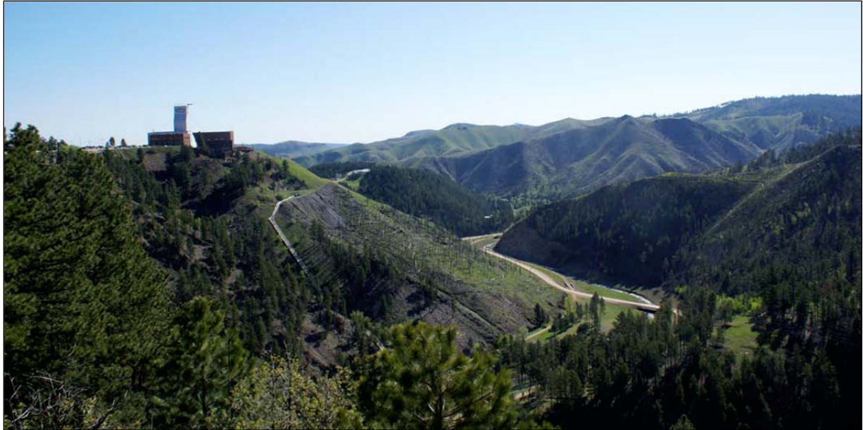
Figure 2-3: Sanford Laboratory Yates Campus shown on the left and Kirk Canyon to the right. [Courtesy of Sanford Laboratory]
