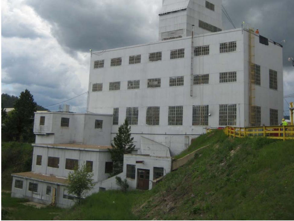
Figure 4-3: Photo of Ross Crusher exterior. [HDR]
