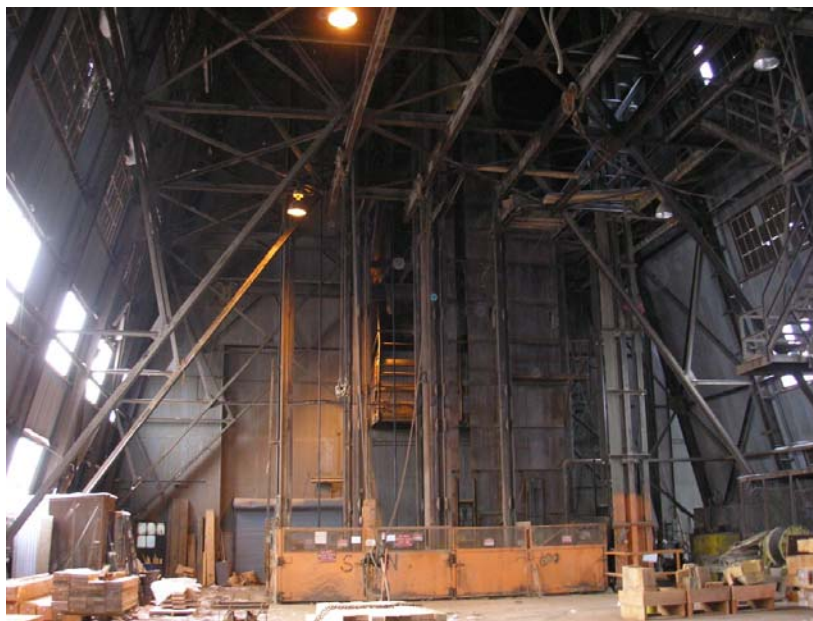
Figure 4-7: Photo of Yates Headframe interior. [HDR]
