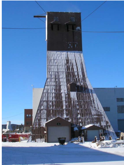
Figure 4-6: Photo of Yates Headframe exterior. [HDR]
