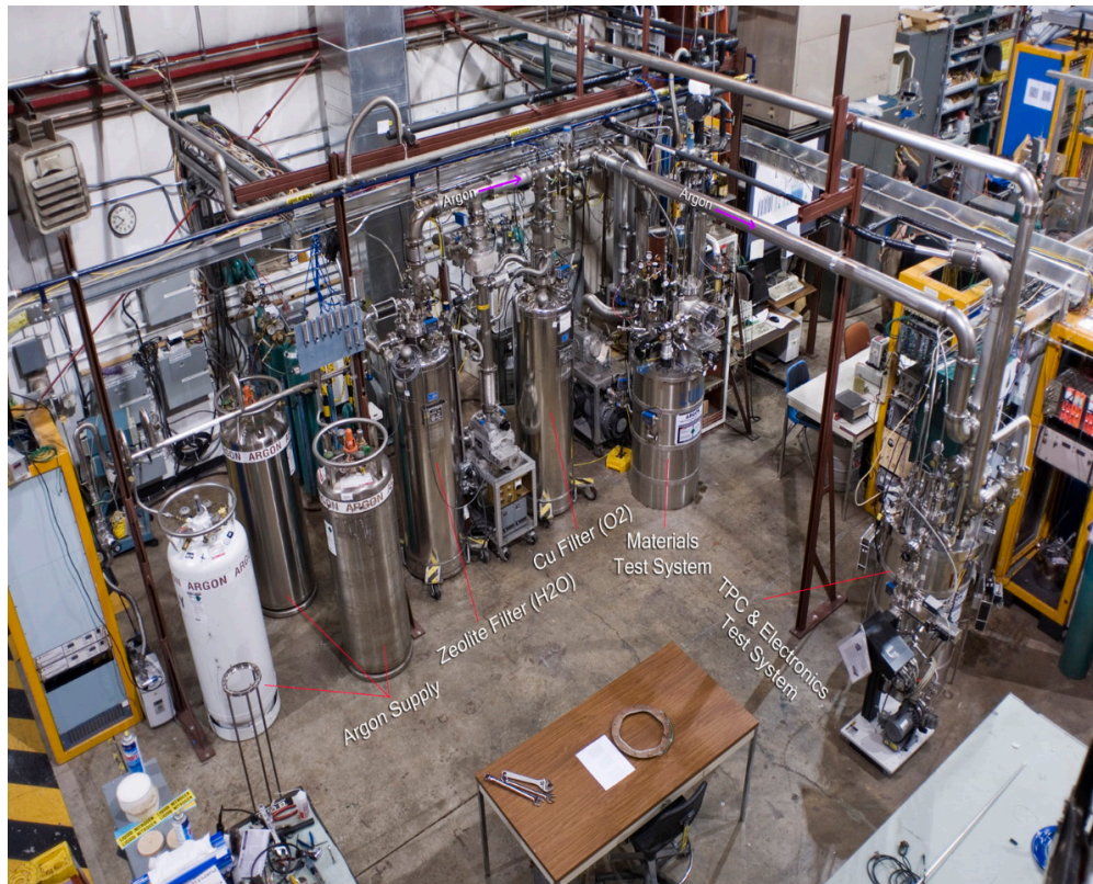
Figure 8-1: Liquid argon area at the Proton Assembly Building at Fermilab
