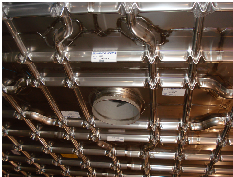
Figure 2-8: Nozzle in roof membrane cryostat (Figure courtesy GTT)
