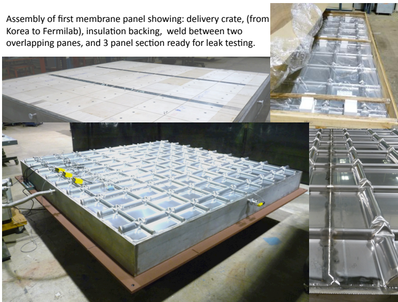
Figure 8-8: Membrane panel assembly and components
