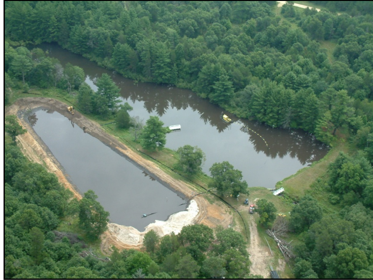
Figure 8. Dredging operations on Hazel Dell Lake.
