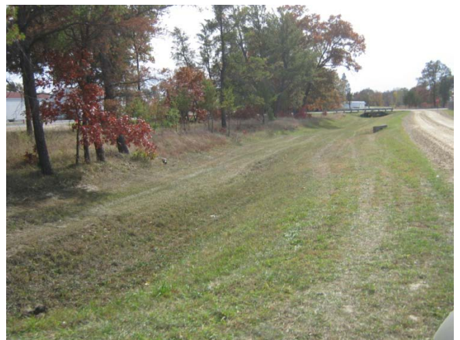
Storm Water Controls-Drainage Ditch west of 13th Ave
