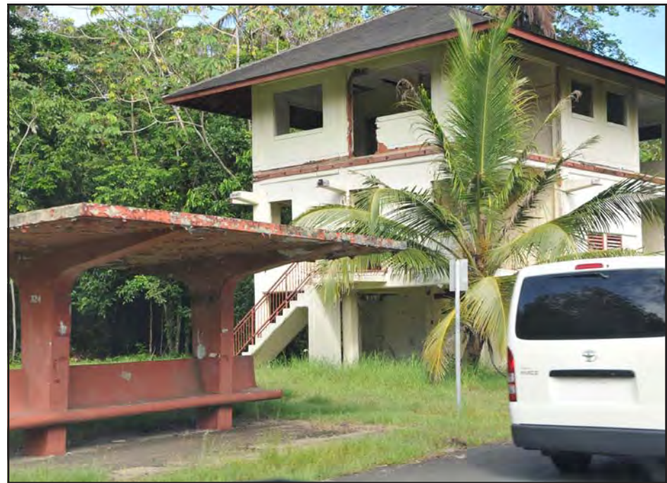
Many of Fort Sherman's buildings have decayed over the years as activity declined. However, the necessity of being prepared for military operations in tropical areas remains as important today as ever.
