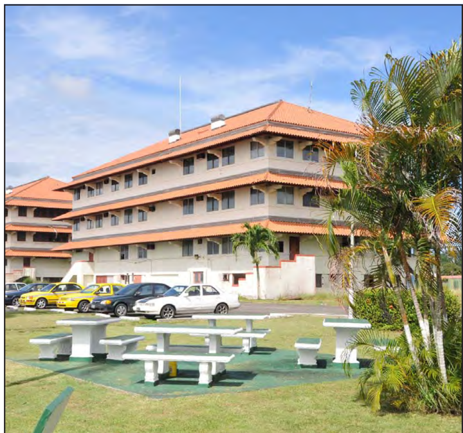
Once a training facility for thousands of Soldiers each year, Fort Sherman consists of more buildings than currently needed for military purposes. The fort originally contained a number of coast artillery batteries operating huge seacoast cannons to protect the Panama Canal.
