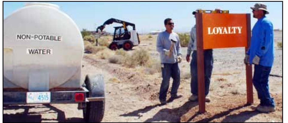
Most recently, maintenance crews were working putting up signs in the Yuma Test Center area.
