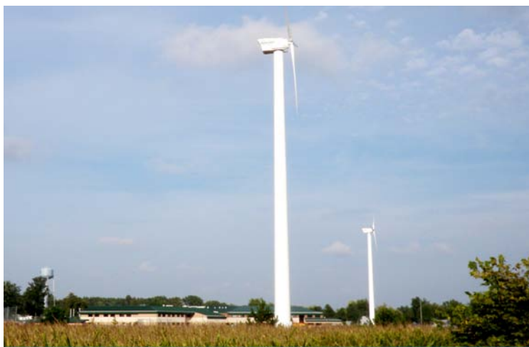
Two 100-kilowatt Northern Power Systems wind turbines provide on-site energy generation for the Upper Scioto Valley School in McGuffey, Ohio. Photo courtesy of NexGen Energy Partners, LLC, NREL/PIX 16741
