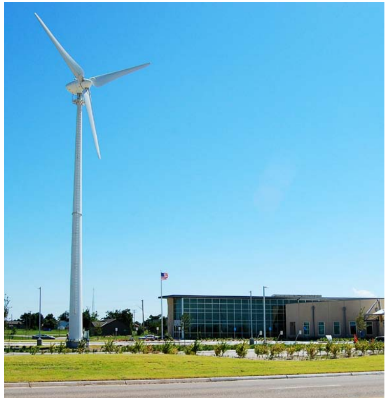
Administrators at Kiowa County Memorial Hospital in Greensburg, Kansas, were so happy with the performance of this 50-kilowatt wind turbine, they installed a second wind turbine on the site. Photo by Joah Bussert, NREL/PIX 17562
