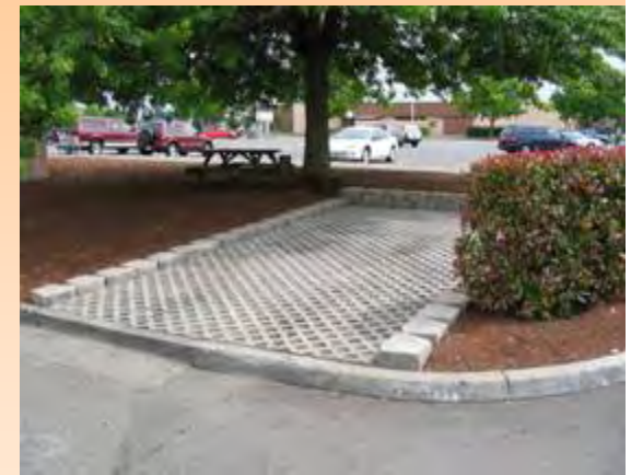
Permeable wash pad
