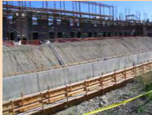
Underground Water Cistern
