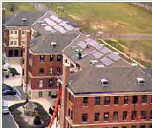
Solar Power at Fort Dix Barracks
