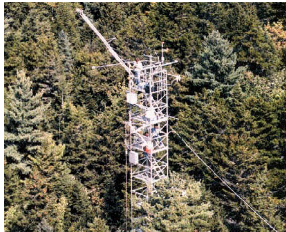
Climate tower at Howland, Maine.
