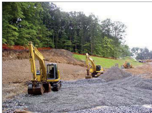
Clearing forest for housing development in Pennsylvania.
