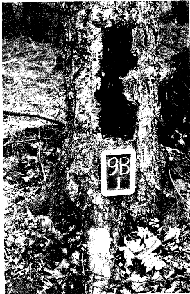
A yellow birch showing stem and root injury from logging. The dark wound face is a good indicator of internal defects. Logging should be carefully done because damage to the butt log can produce considerable loss.
