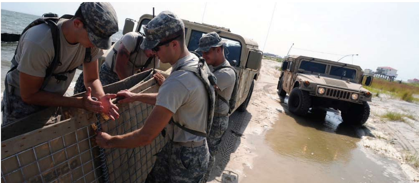
Building and maintaining miles of HESCO barriers to protect Dauphin Island, Ala., beaches. Photo by Staff Sgt. Jim Greenhill
