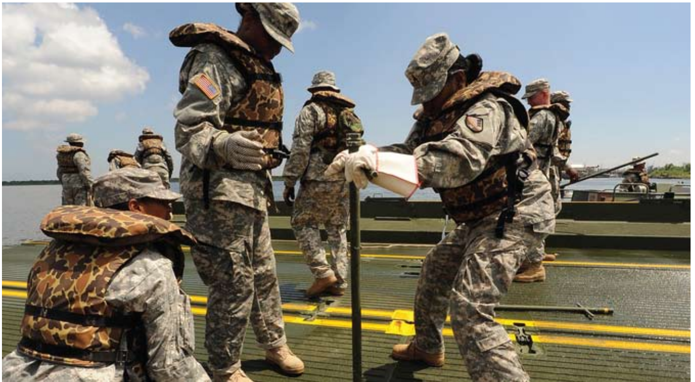
Constructing a 300-foot temporary wharf. Photo by MSgt. Toby M. Valadie
