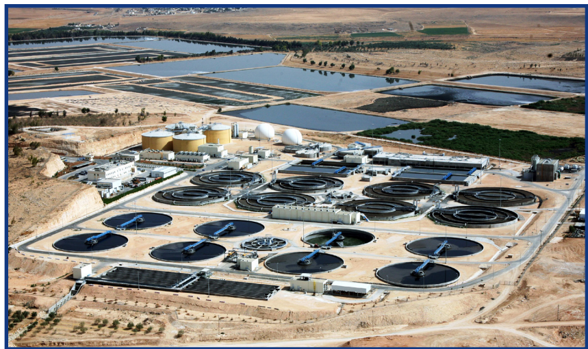
An MCC grant of $93 million is supporting the expansion of the As-Samra wastewater treatment plant as part of a public-private partnership.
