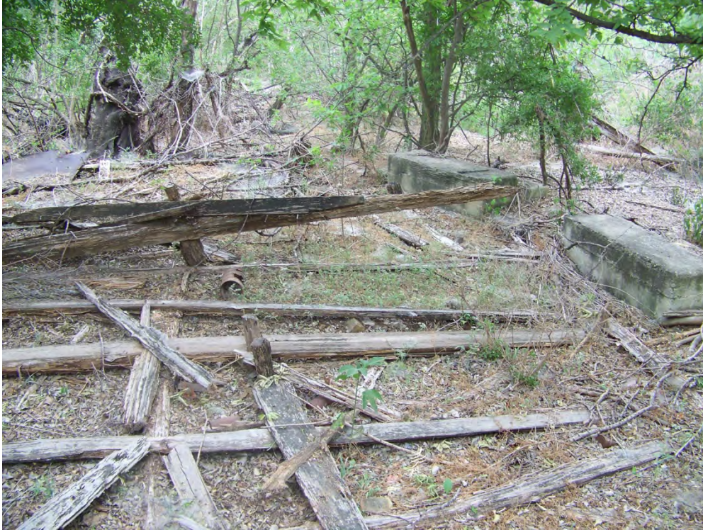
Figure 19. Remnants of collapsed structure at 41BX1886, looking south.
