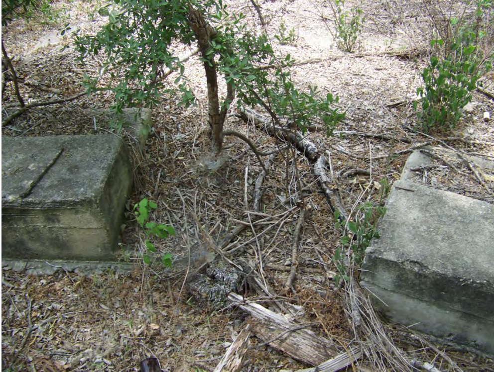
Figure 21. Dual-step concrete porch at western edge of collapsed structure, looking down.
