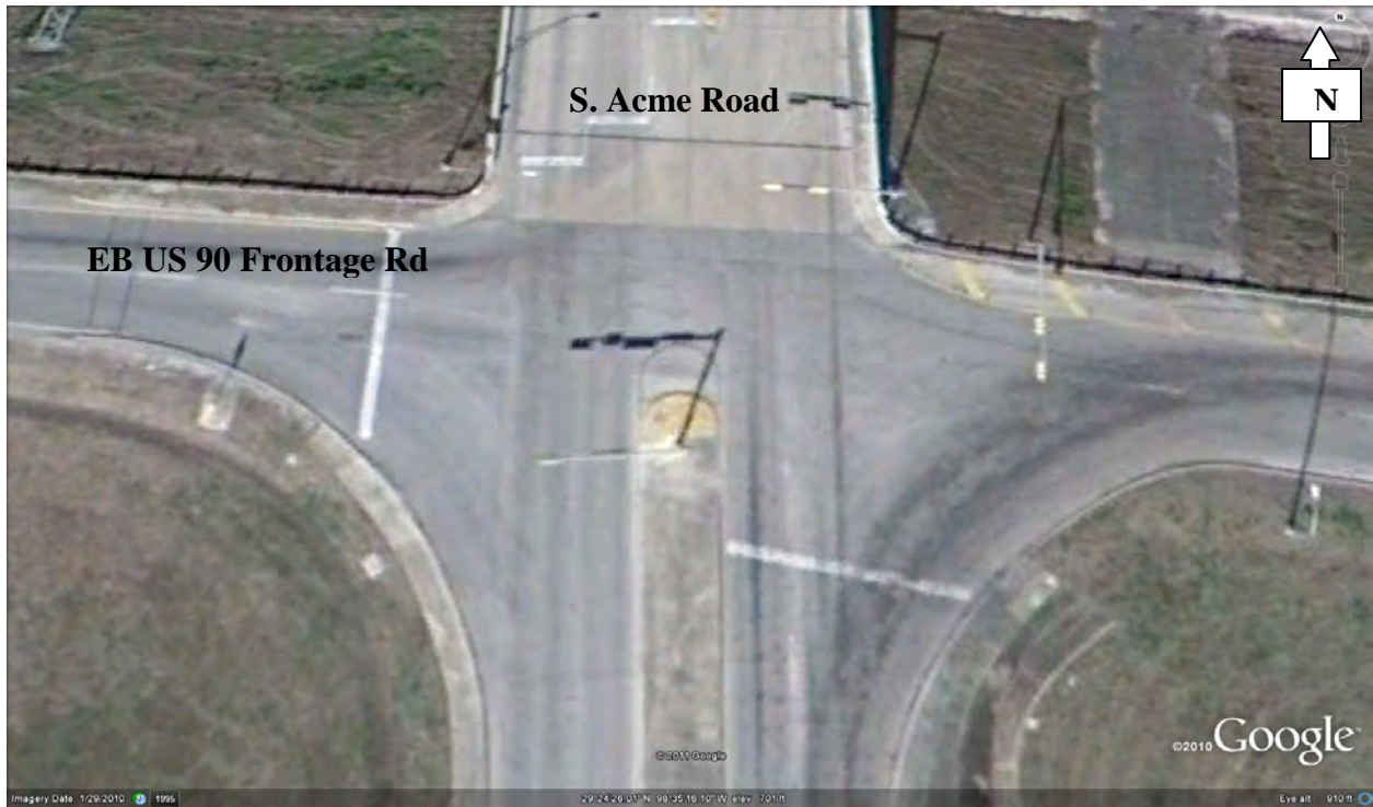
Figure A5. S. Acme Road at East Bound US 90 Frontage Road
