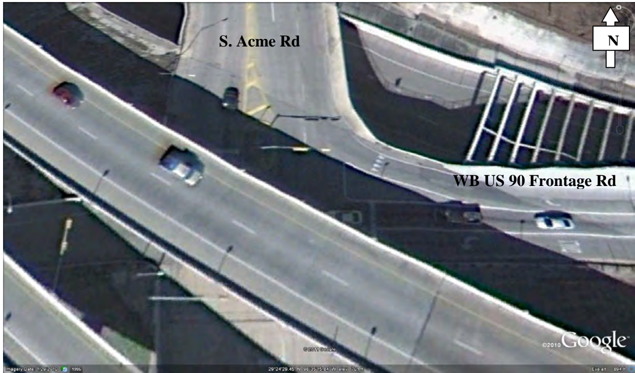
Figure A6. S. Acme Road at West Bound US 90 Frontage Road
