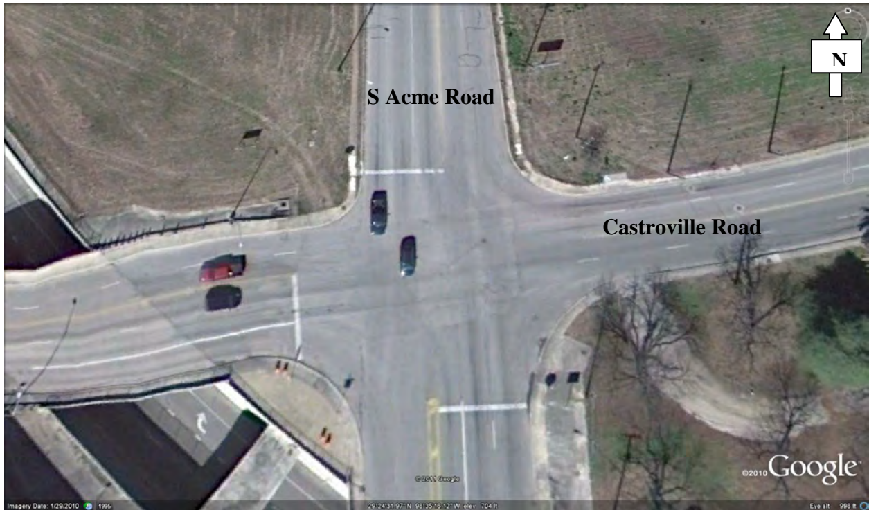
Figure A4. Castroville Road at S Acme Road
