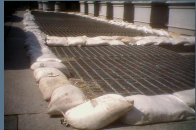
WMATA vents with one layer of sandbags prior to Federal Triangle Stormwater Study (above) and increased protection using the Study's predicted ponding levels (below)
