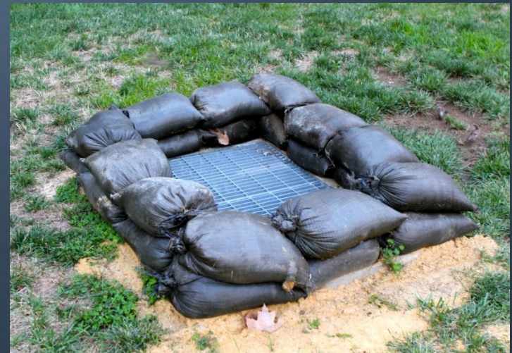
WMATA vents with one layer of sandbags prior to Federal Triangle Stormwater Study (above) and increased protection using the Study's predicted ponding levels (below)
