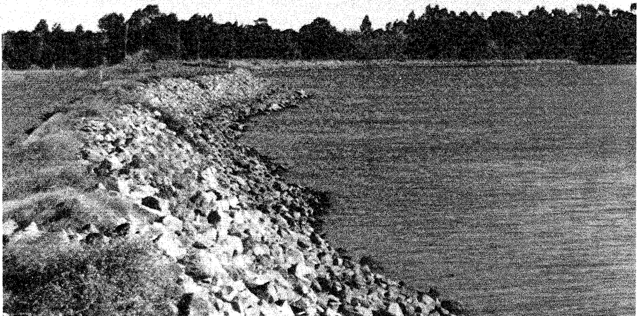
Figure 4. Project levee on north fork of Mokelumne River. Note absence of riparian or emergent vegetation.
