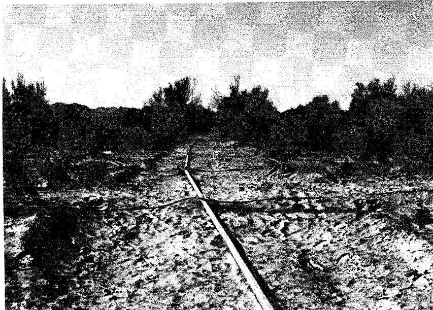
Figure 39A. Above-ground drip irrigation is the least expensive and most efficient means for watering trees. Special care is needed for tracking duration and amount of irrigation on trees and shrubs in accordance with physical parameters. Photo from Cibola National Wildlife Refuge (1979) by J. Disano.
