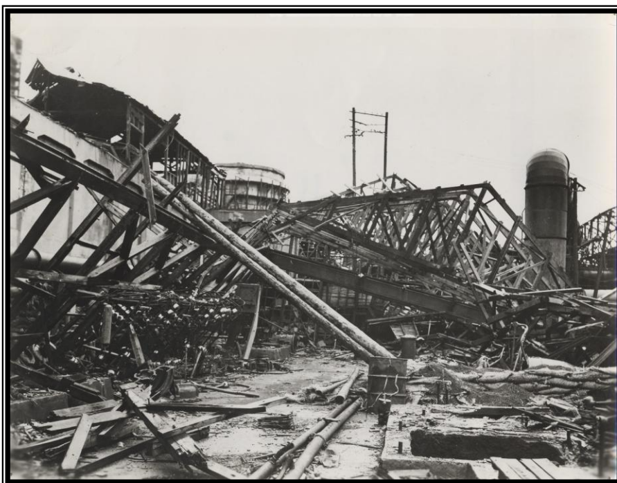
Figure 6. Remains of North Korea's largest ore smelting facility in Chinnampo, North Korea following a visit by the 22d's B-29s in 1950.
