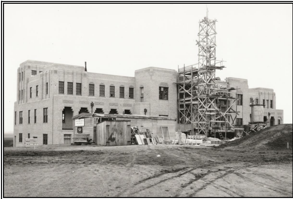
Figure 11. Construction of the Wichita Municipal Airport early 1930s (Kansas Aviation Museum).
