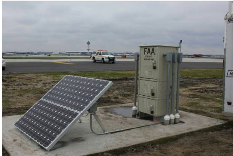
Figure 10: Site Installation at JFK
