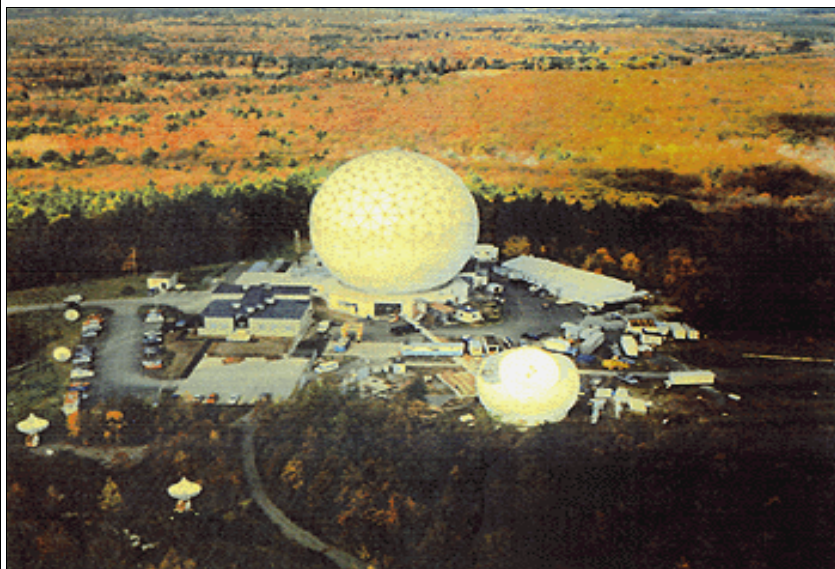
Haystack (background) and HAX (foreground) radar domes are NASA's main source of data for debris in the size range of 1-30 cm.
