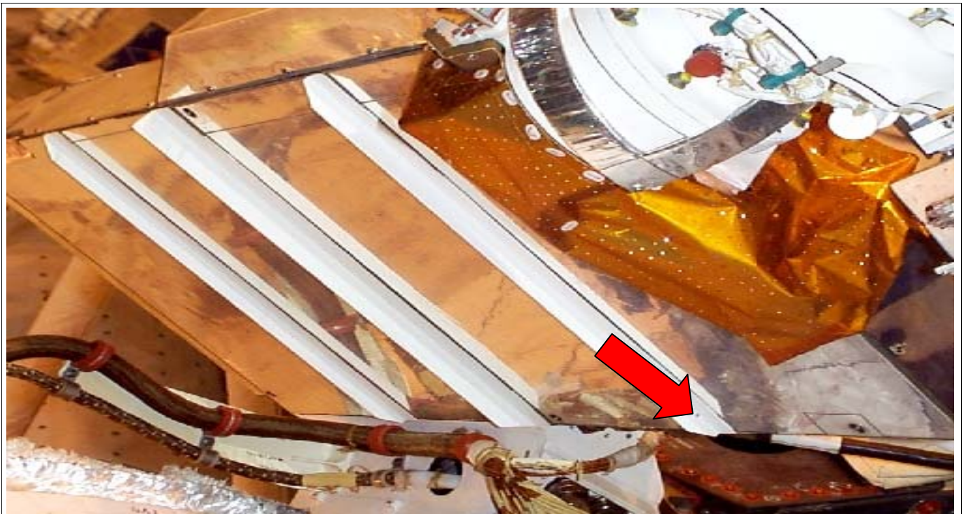
Location of the impact crater on the Ku-band antenna electronics box of OV-102.
