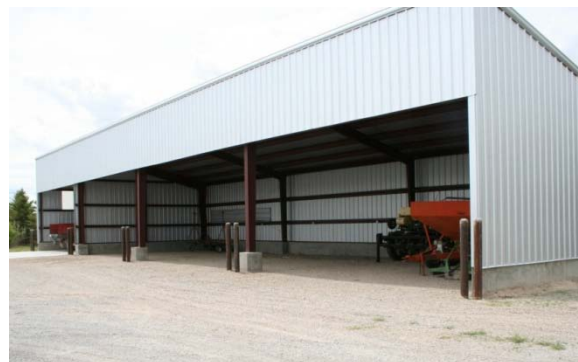
The new PMC equipment barn.
