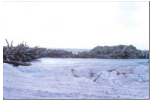
Figure 295. These trees were cleared for the construction of the Majuro airport (Photo: James McVey).
