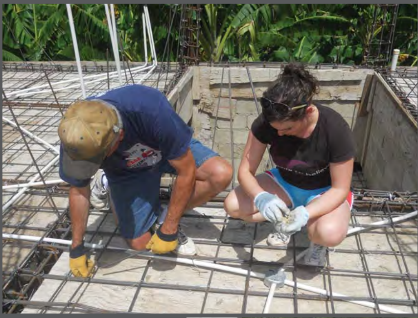
Mike Gomski and daughter Vicky building a rooftop
